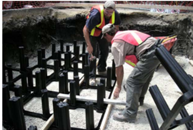
Installing Silvacell to increase soil volume for urban trees
