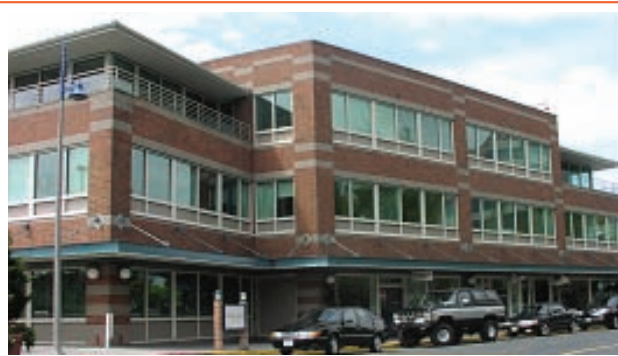
Figure 9. Use of building modulation, window patterns, brick, balconies and awnings help lend this building a human scale.
