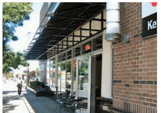
Figure 31. Building-mounted lighting is encouraged to enhance the pedestrian environment
