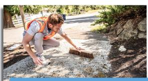
With proper maintenance, a typical permeable pavement system has a life span of approximately 25 years.
