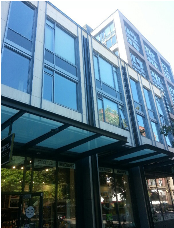
Upper levels set back from base at western edge of office building; ample glazing and canopies enhance pedestrian experience
