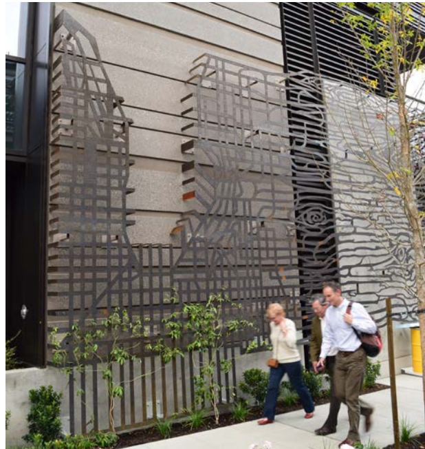
Vegetation, art, and screening provide visual interest at blank walls (center image 4)
