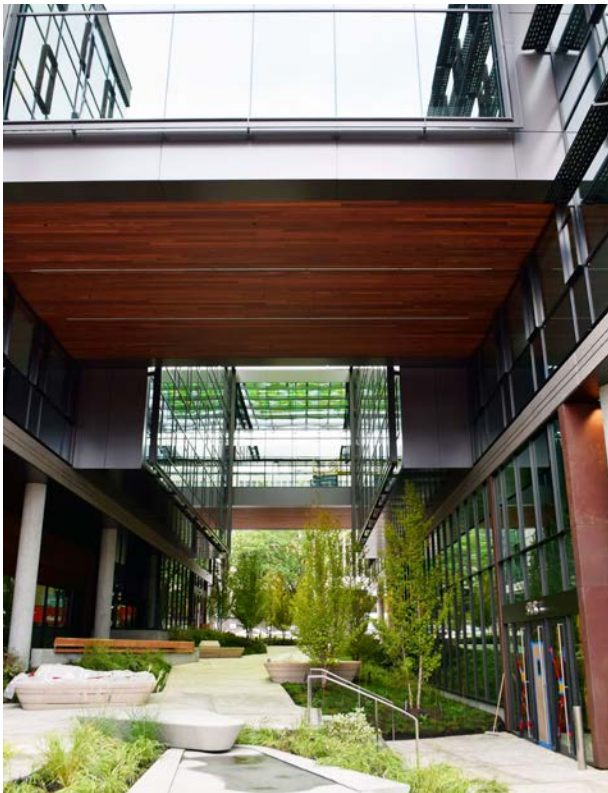
Two-story pedestrian pass-through to promote physical and visual connections, and to reduce apparent building bulk at grade level
