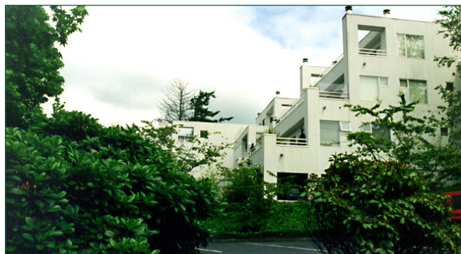
mmTerraced buildings reflect the hillside topography ringing Kirkland's Downtown.
